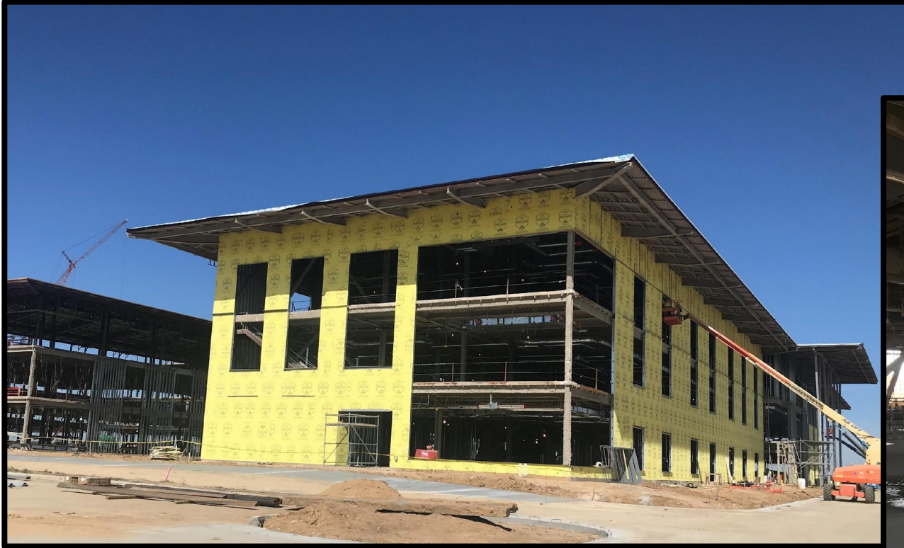
Exterior with insulated sheathing in Area A
